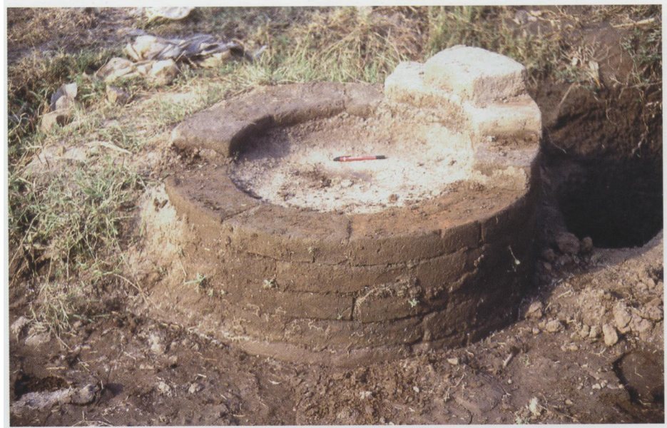
Fig. 13: Brick-lined well in process of being dismantled for building material.
